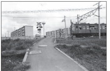
A train passing through the crossing of Nambu Line The Yagawa-kita housing complex was rebuilt. A scene from around 1968 Owned by Kunitachi Local Culture Museum
